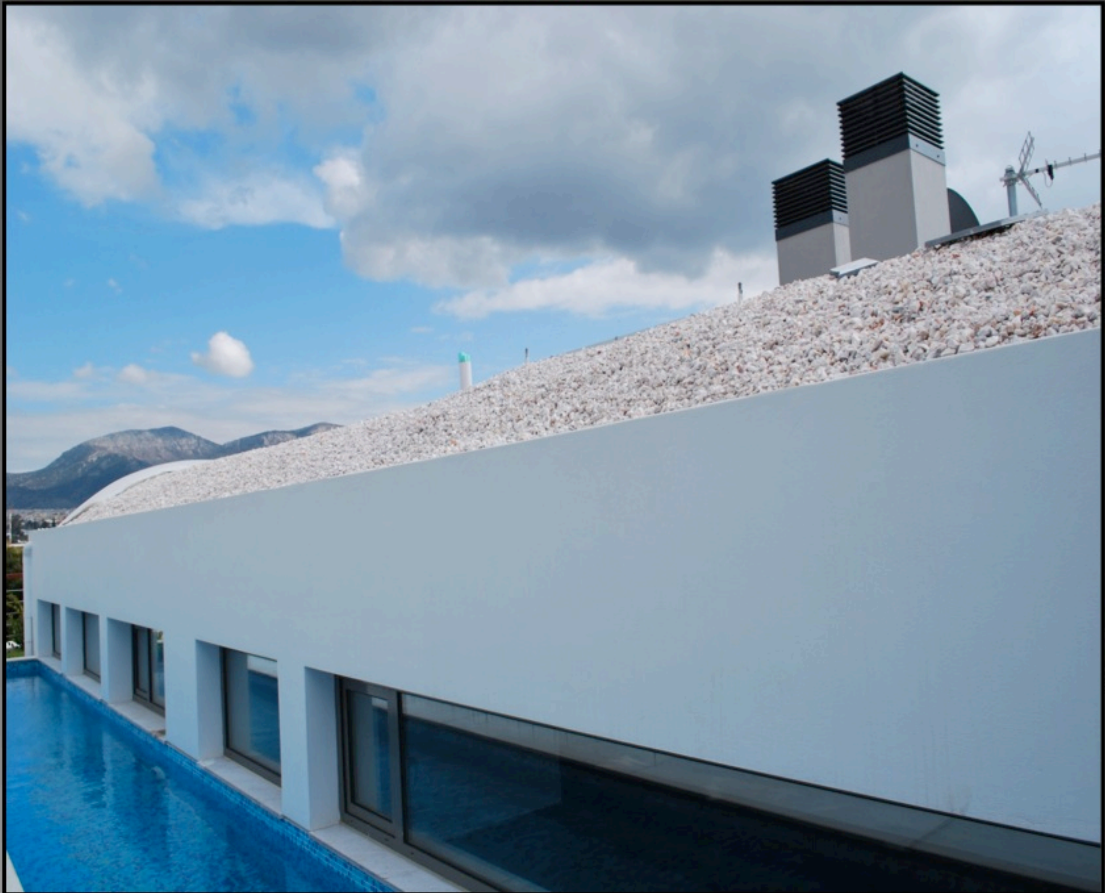
Side view of swimming pool , on the 4 th Floor
